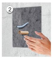
Place the cuff over the water and power connection. Press the cuff firmly onto the wall.
