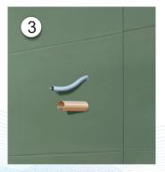
The tile adhesive can be applied directly to the sleeve and you can tile the wall immediately.
